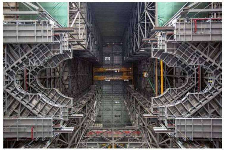
High Bay 3 inside the Vehicle Assembly Building at NASA's Kennedy Space Center in FLorida. The newly installed platform will complete the second of ten levels of work platforms that will surround and provide access to the SLS rocket and Orion spacecraft for Exploration Mission <sup>1</sup>
